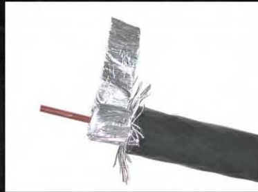
If tri-shield or quad, remove outer layer of foil
